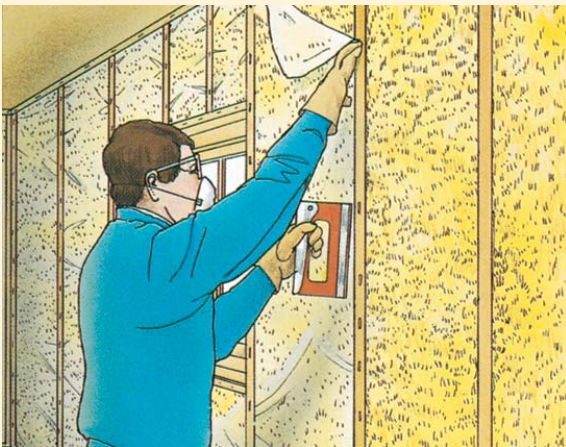
INSULATING EXTERIOR WALLS: Knauf unfaced blankets can be used with a polyethylene vapor retarder.
