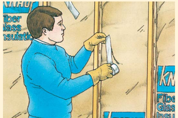
Patch any tears in vapor retarders.
