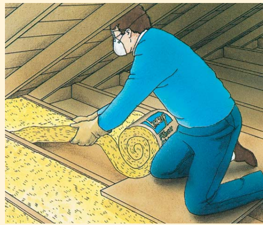
INSULATING WITH FACED INSULATION: Keep the vapor retarder down, toward the “warm-in-winter” area of your house.
