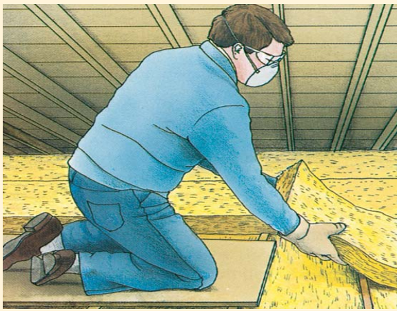
INSULATING WITH UNFACED BLANKETS: Begin laying the blankets at the outer edges of the attic and work toward the middle.
