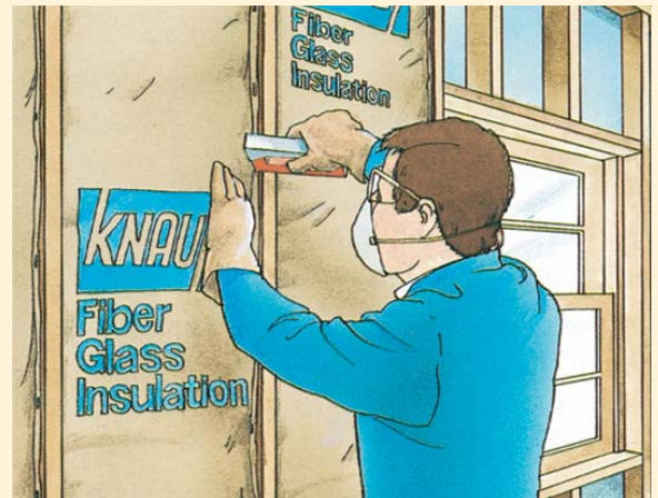
INSULATING EXTERIOR WALLS: The location of the vapor retarder is recommended toward the inside of the home.
